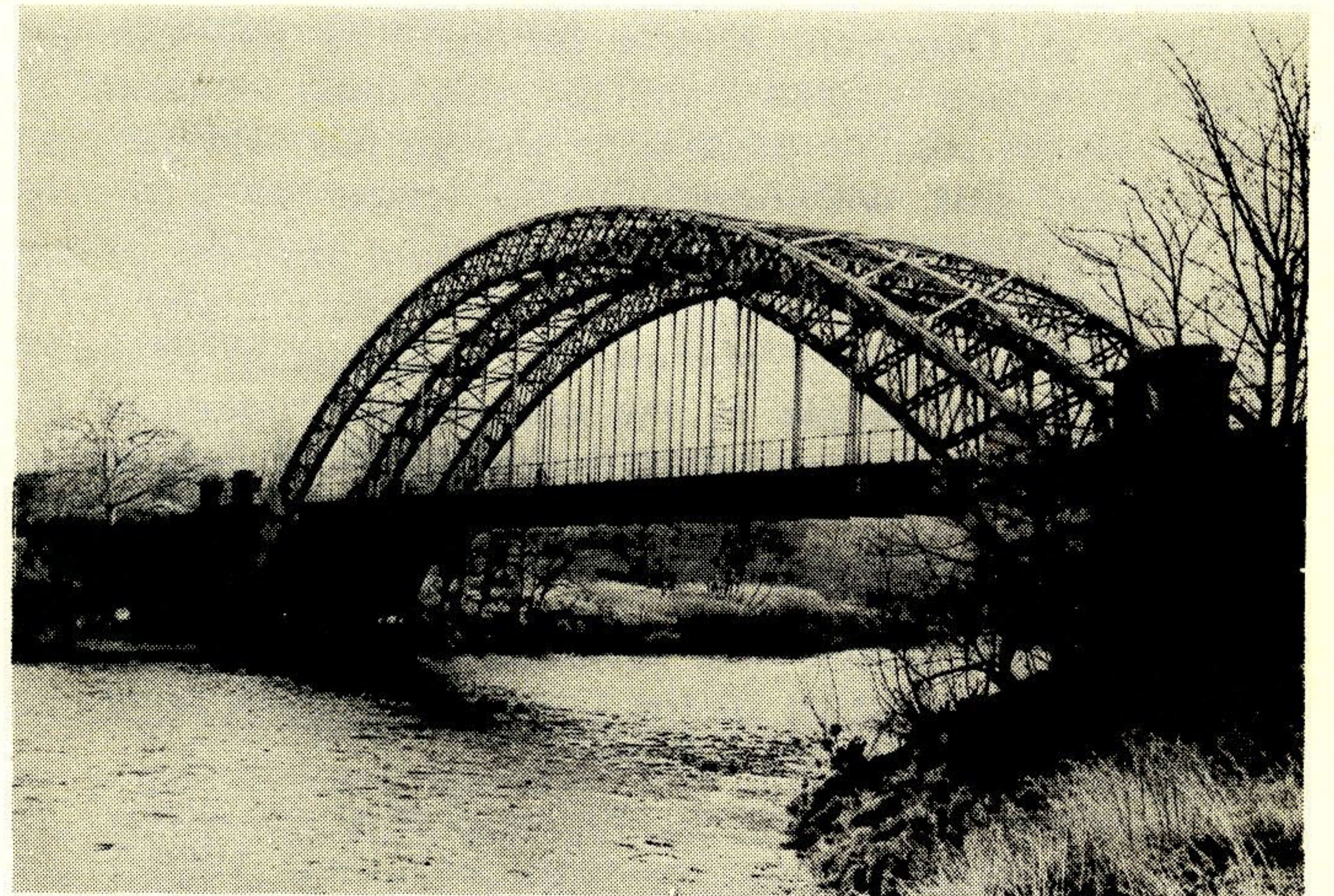
One hundred years old this month—the fine railway bridge over the Tyne at Hagg Bank was opened in October, 1876—to complete the Scotswood-Newburn and Wylam Railway. It cost £16,000 to build and is now being given a commemorative coat of paint by the County Council.
