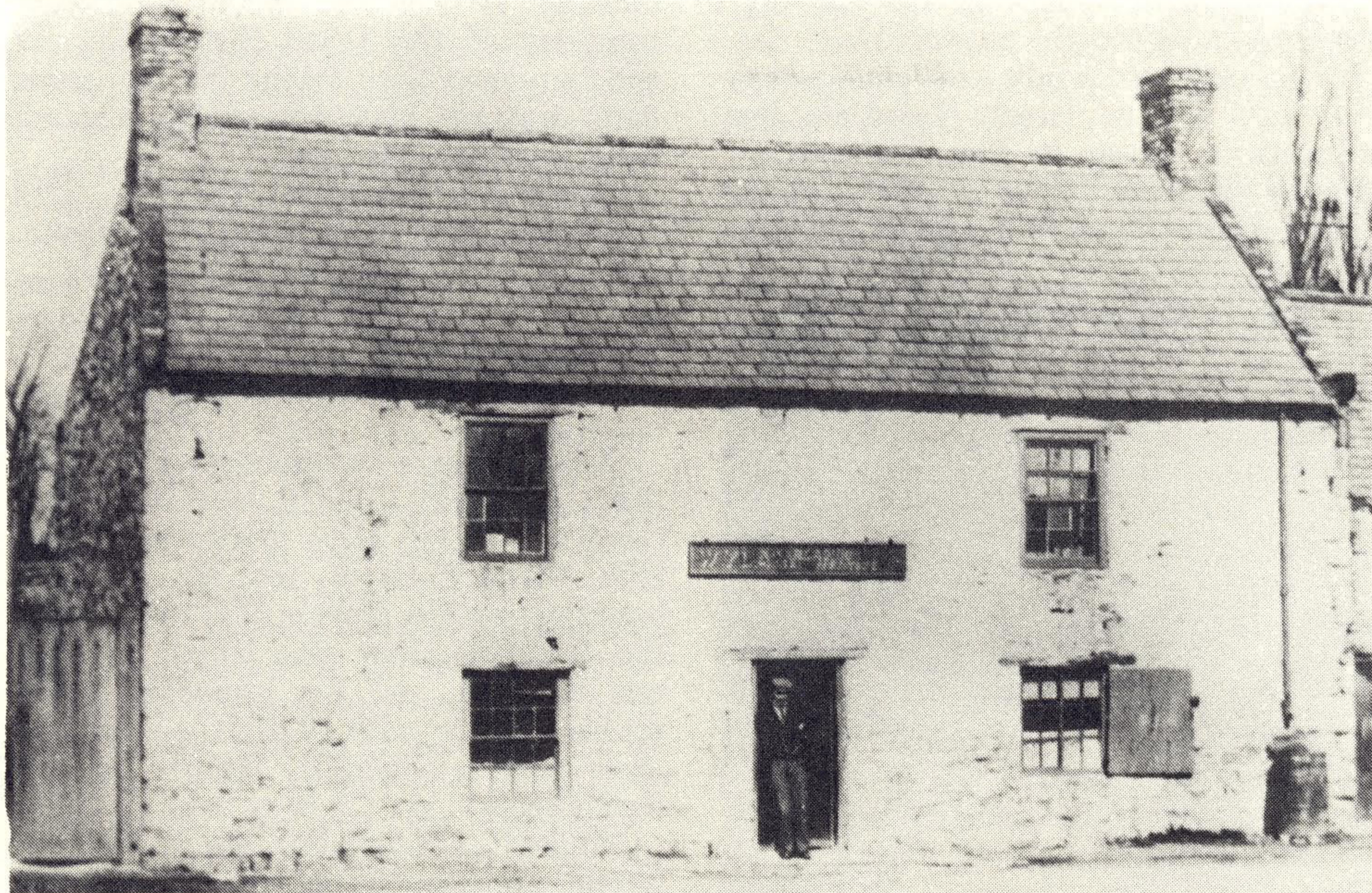
Hardly big enough for Community Week activities today! This was the old Institute used until the 1890's when the present building was erected. It stood on Charlie's Corner and was demolished in the 1920's.
