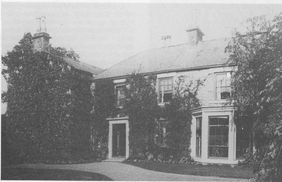
Wylam Cottage—a view of the south front as it was c. 1900.
