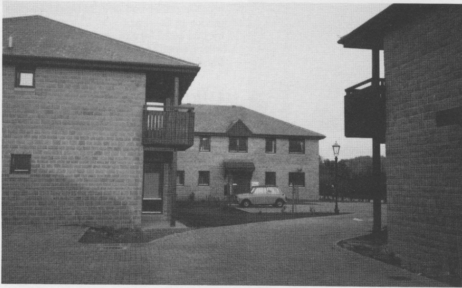
Changing landscape — work on the new Stephenson Court flats is now completed.
