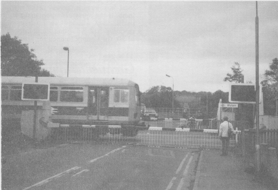
Full barriers down at the Wylam level-crossing on a quiet Sunday afternoon, safely and effectively preventing access onto the railway. Compare this with the photograph elsewhere of the crossing at Stella which only has half-barriers.
