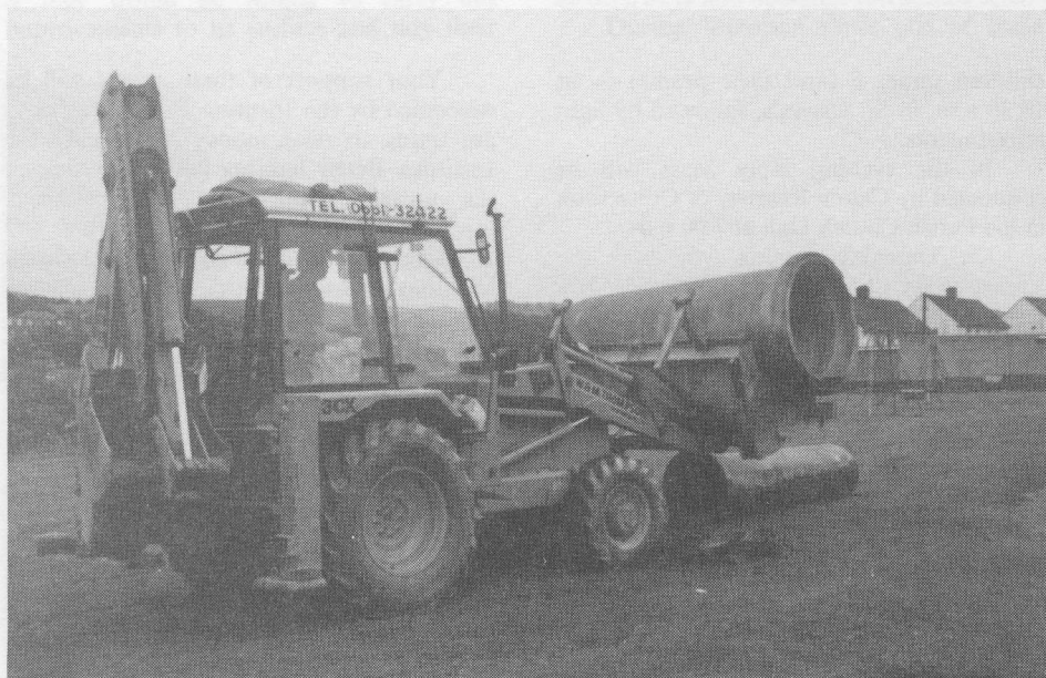
Following several complaints the old concrete pipes have been removed from the Hedley Road playground — in the interests of safety.
