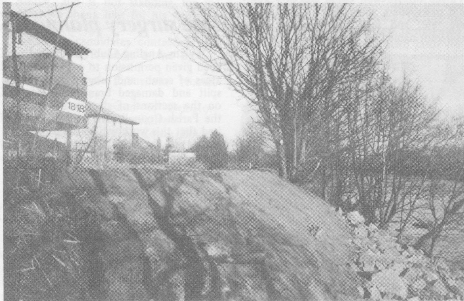
When the surface-water outfall on Stephenson Terrace was replaced earlier this year, the riverbank was also strengthened with boulders to reduce future erosion. Trees have now been planted on the banktop.
