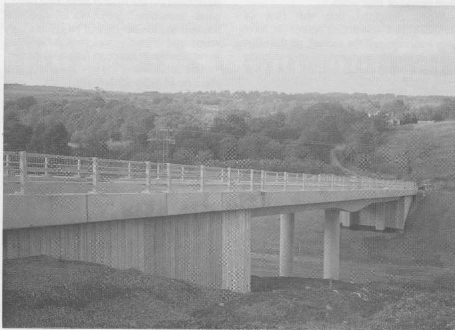
The new bridge carrying the Hagg Bank - West Wylam road over the Prudhoe By-pass. This is the last major structure to be completed. The new bridge is now open to traffic and construction of the section of by-pass beneath it is in progress.
