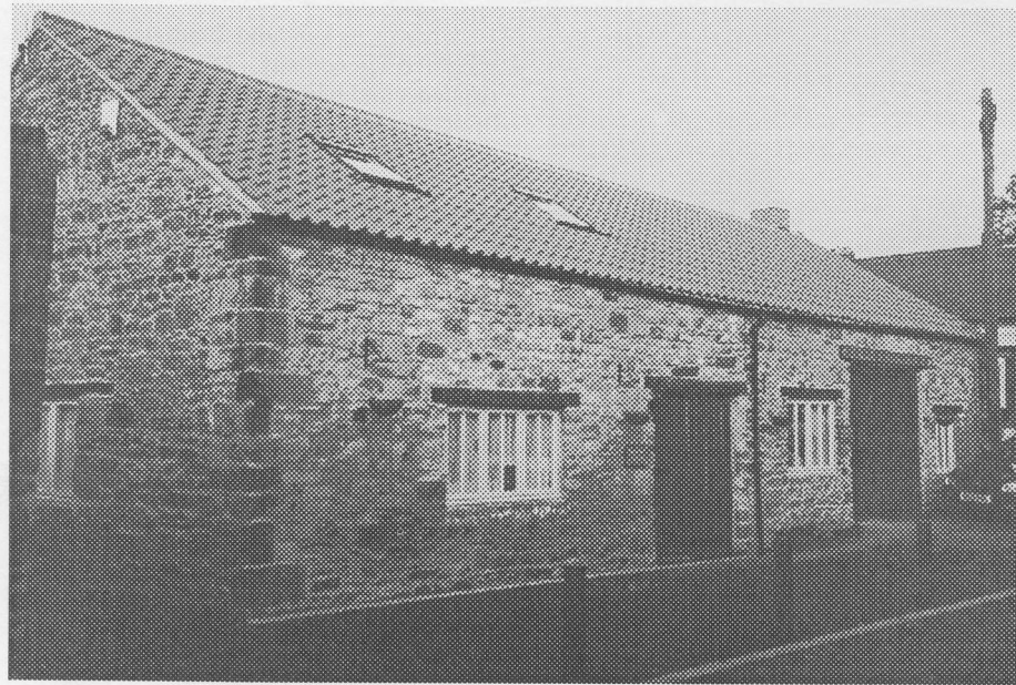
The old blacksmith's forge, previously part of the Wylam Colliery workshops in West View, which was attractively converted into a cottage and tile and craft workshop for Debbie Conley last year. Congratulations to all involved in this scheme, which has greatly improved this corner of the village.
