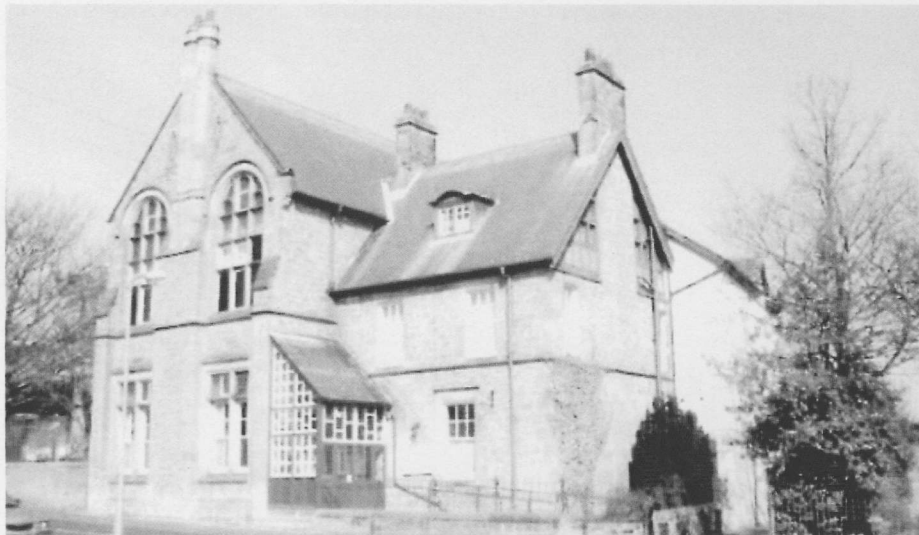
The village Institute and Community Centre looks in fine condition in this recent photograph, but closer inspection has shown that various external repairs will be necessary soon.
