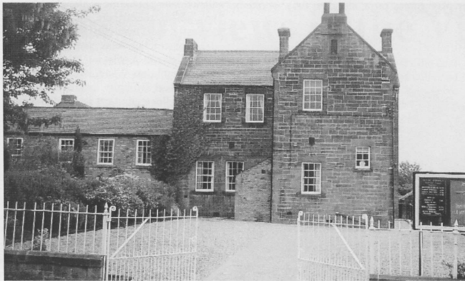
The Brethren have recently created an attractive access and parking area to their premises on Woodcroft Road, in keeping with the tradition and character of the old school buildings, which will be 150 years old next year! A special birthday celebration in 2004?
