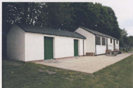
The new pavilion extension
