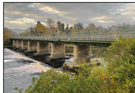
Wylam Bridge - Work is now set to commence in January
