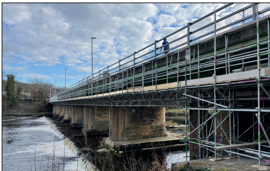
Scaffolding surrounds Wylam Bridge, as re-painting work continues
