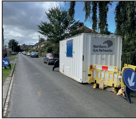
Work in progress on Woodcroft Rd in early October
