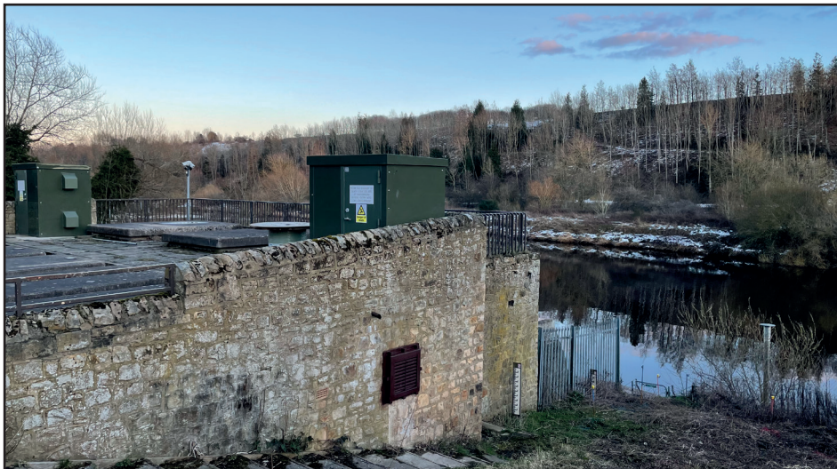
New Eel Screens will be installed at Ovingham Pumping Station, starting in March 2023
