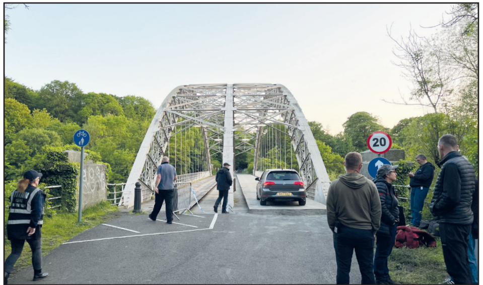
Points Bridge was used extensively during the shoot, with a special platform added to enable cars to access the bridge deck
