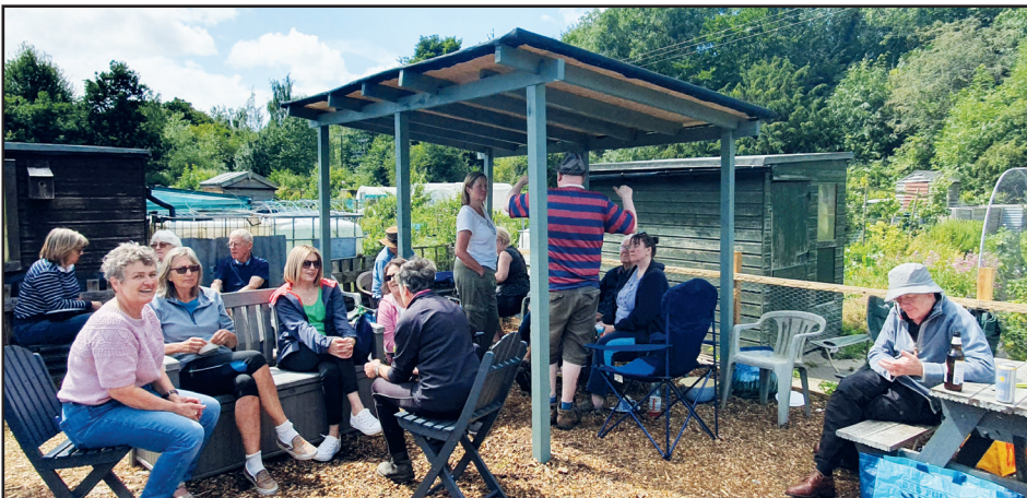
The new shelter has been built in the central communal area of the allotments
