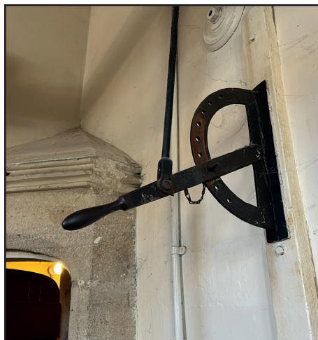
A lever to pull back the clock chime hammers while the bells are being rung
