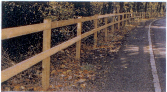
A section of the finished fence
