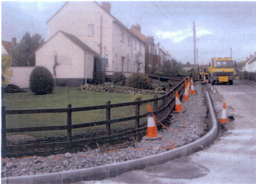
Work in progress in Hackworth Gardens
