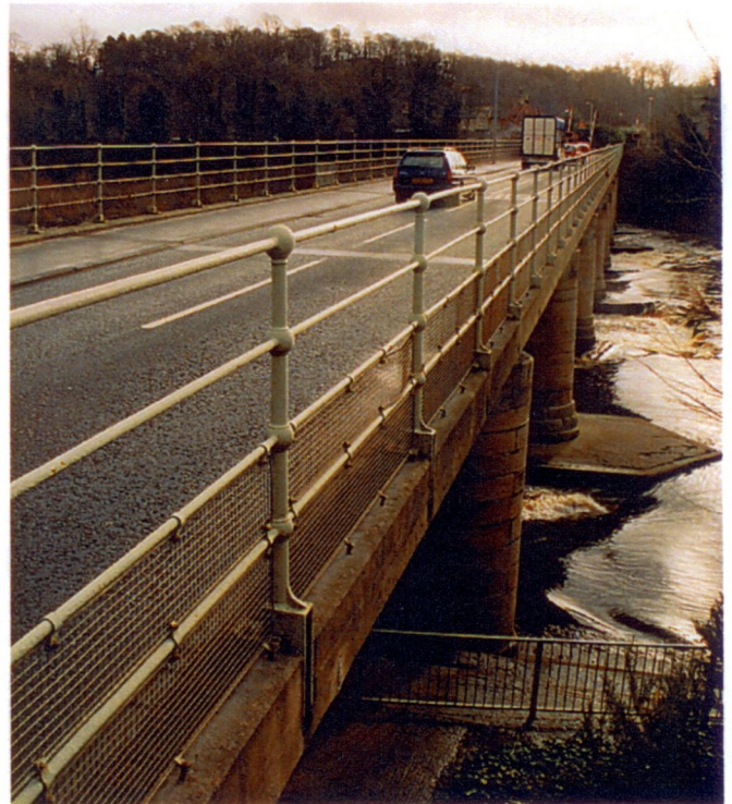
Wylam Bridge - soon to undergo major changes
