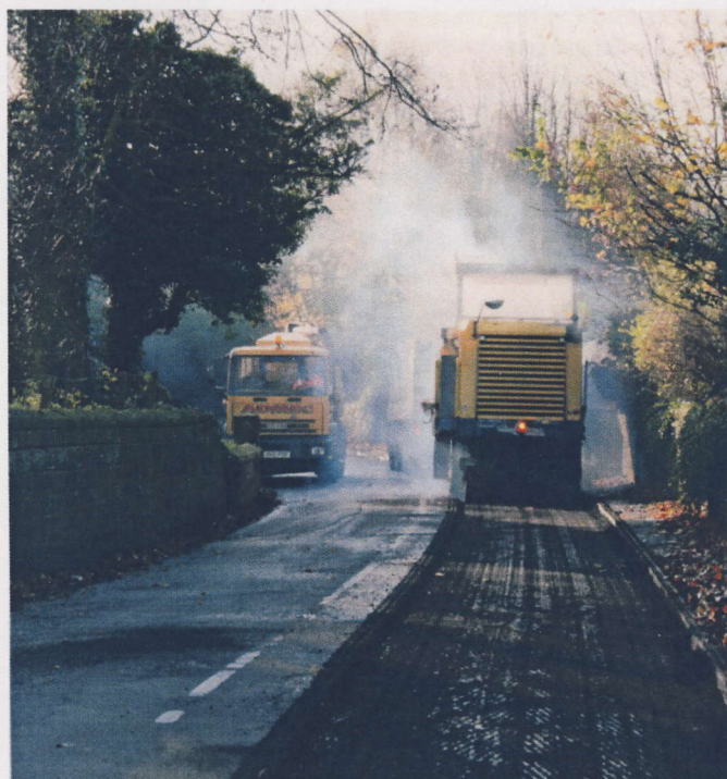
Road-planing operations on Holeyn Hall Road
