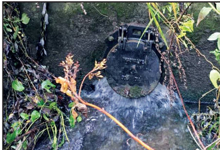
A sewer overflow emptying into the River Tyne
