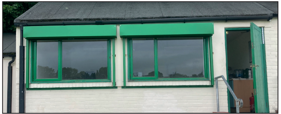
New electric shutters are in place at the pavilion
